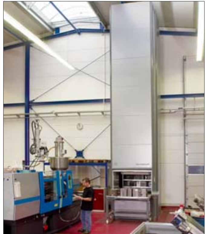
In this injection molding facility, a vast amount of floor space was freed up by storing tools in a Hänel Lean-Lift®
